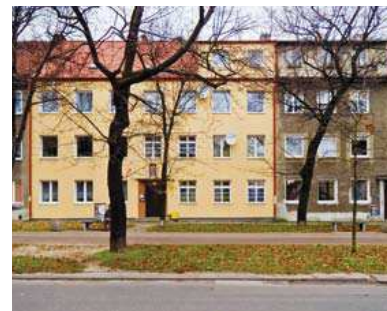
Fig. 4.22 Renovation wrongdoings: painful lack of window bars in a newly renovated tenement house in Wrzeszcz (above) and unintended (?) 'disneyfication' of a facade in Nowy Port (below) Authors: Piotr Połoczański and Izabela Sitz-Abramowicz (Wolne Forum Gdańsk 2010)
